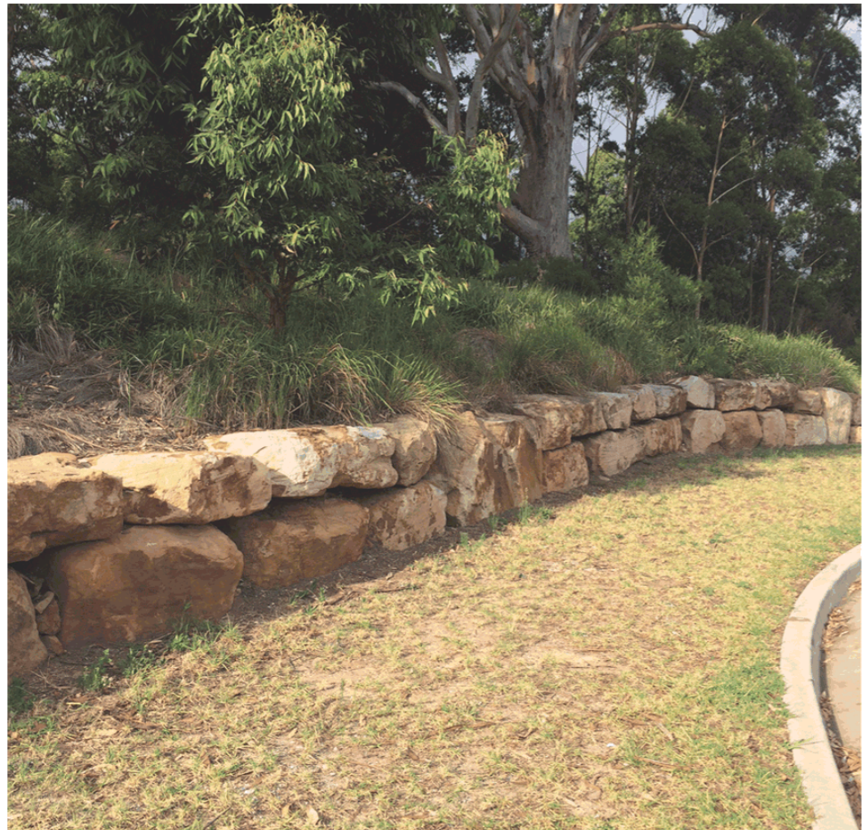
Retaining Wall, Bulli
