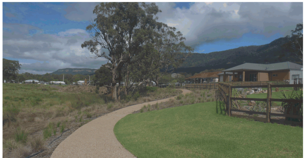
Concrete pathway adjacent to riparian area, Wongawilli
