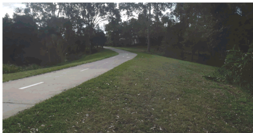
Urban greening and stormwater management, Nyrang Park, Keiraville. A good example of pathways located at top of bank in open space
