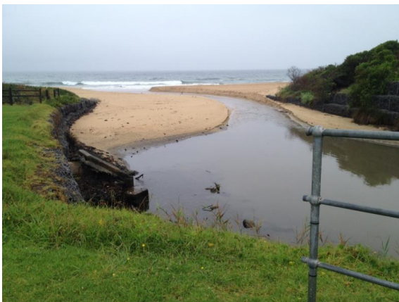
Plate 19 Open entrance after heavy rain (WCC 11/1/2015)
