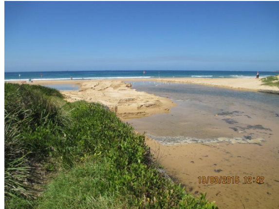
Plate 23 Entrance following 2015 works (WCC 19/3/2015)
