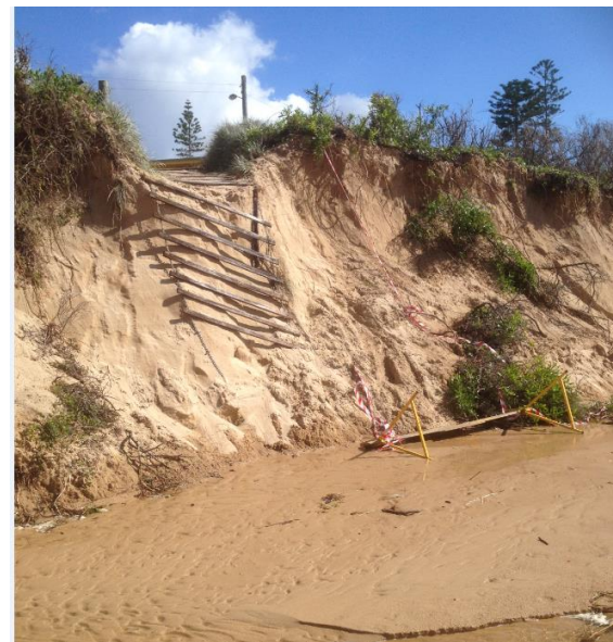
Plate 4 Damaged beach access (WCC 27/12/2013)
