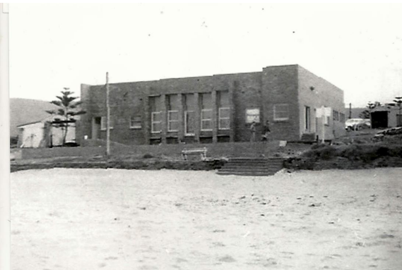
Plate 6 Sandstone wall and steps 1958 (Bulli SLSC)
