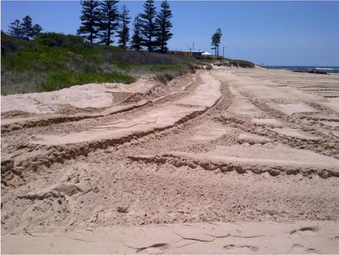
Plate 21 Reshaping of beach/ dune following entrance scour (WCC Feb 2014)
