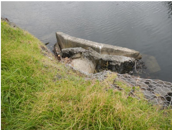
Plate 14 Stormwater pipe headwall
