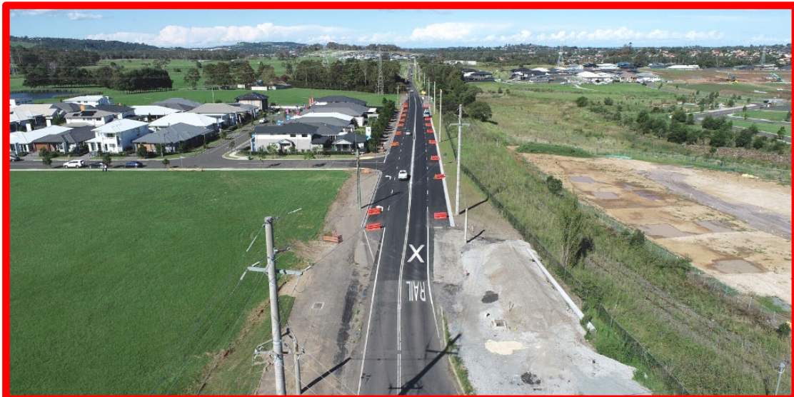
West Dapto Road Upgrade Works (Stage 1B) – April 2023.
