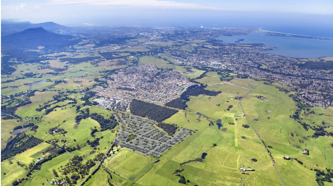
Figure 1 WDURA – aerial view looking north east
