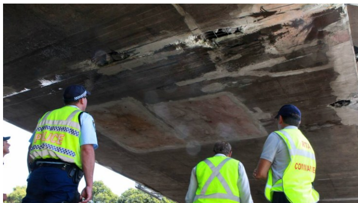
Figure 36: University Avenue is 4.9 m for northbound traffic, but only 4.6-4.8 m for southbound traffic. It has been stuck by oversized vehicles several times, including as recently as 2018. (Humphries, 2015)
