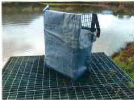
Image 4 Outlet trash basket wrapped in geofabric
