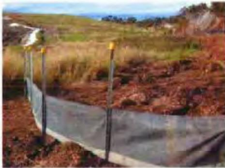
Image 2 Extra sediment fence installation
