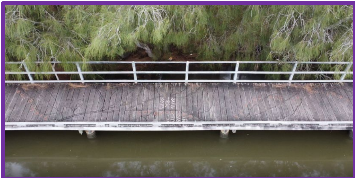
Hooka Point Berkely, work commenced on replacing the ageing timber deck of the jetty and footbridge as well as working with artists to repair and maintain as many of the existing artworks as possible.
