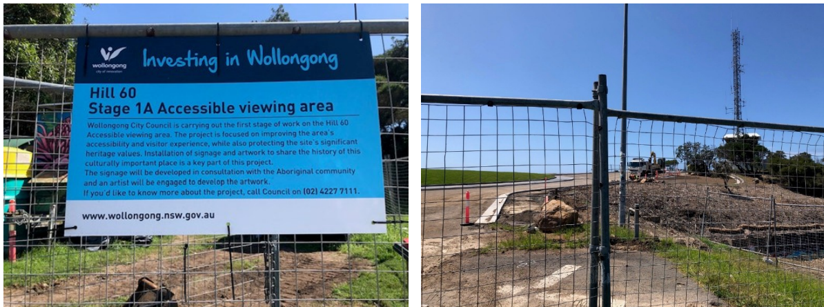
Figure 4 Site Visit Photographs 2024 Accessibility and Viewing Area Upgrade Capital Works Project
