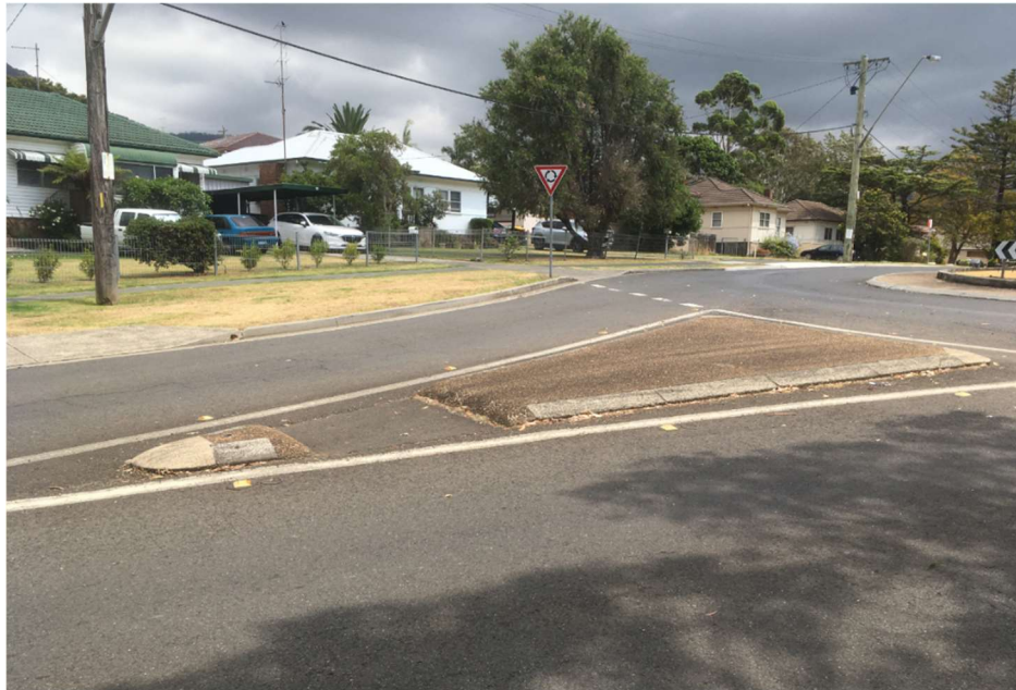
Gap in traffic island is too small to accommodate wheelchairs, prams or bicycles
