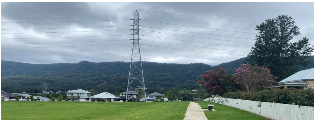
Figure 18 Site elevation of the high voltage powerline running north-south within Stane Dyke Park
